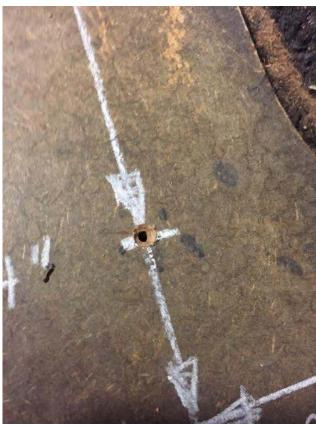
4. Now use the bracket as a template for the second hole as in the photos. Remove the bracket after drilling.
